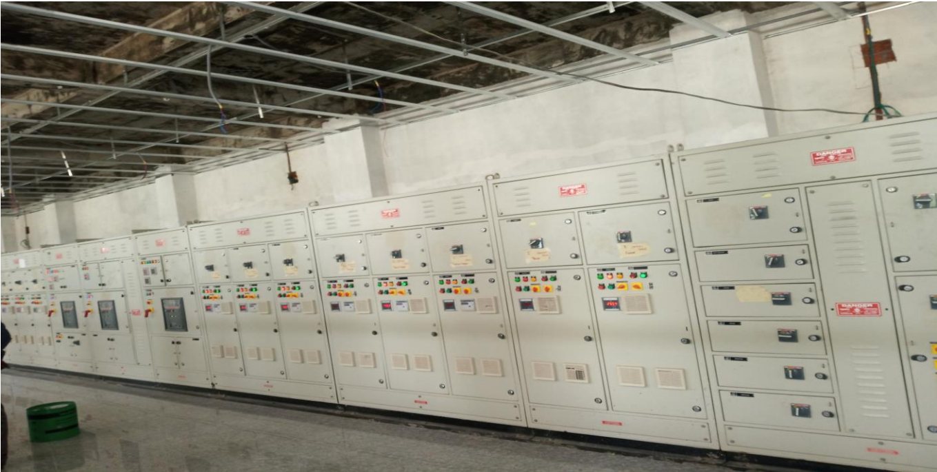
Electrical Mains for the operation of pumps:
